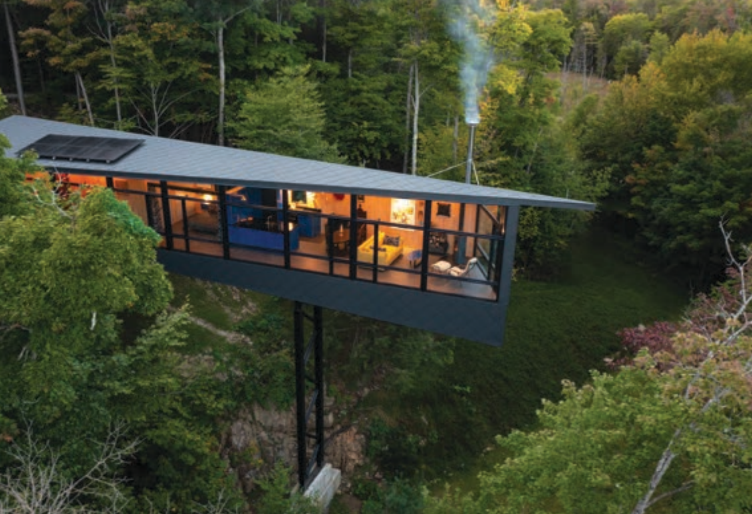
GREEN HOUSE Kariouk designed the cabin with eco-friendly fixtures, including bat pods and rooftop solar panels
