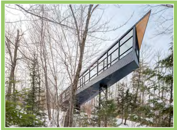
A 60-foot tall steel mast supports the cabin, which is designed in a way to allow for a 25-foot cantilever. Photo courtesy Scott Norsworthy
