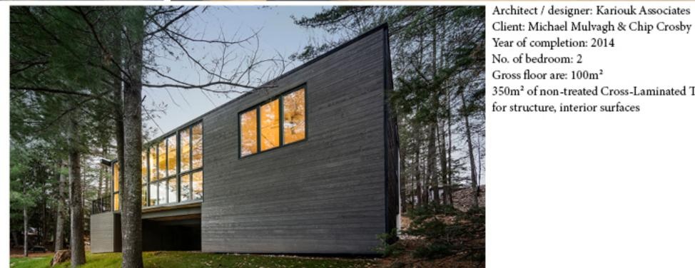
Client: Michael Mulvagh & Chip Crosby Year of completion: 2014 No. of bedroom: 2 Gross floor are: 100m² 350m2 of non-treated Cross-Laminated Timber (CLT) used for structure, interior surfaces
