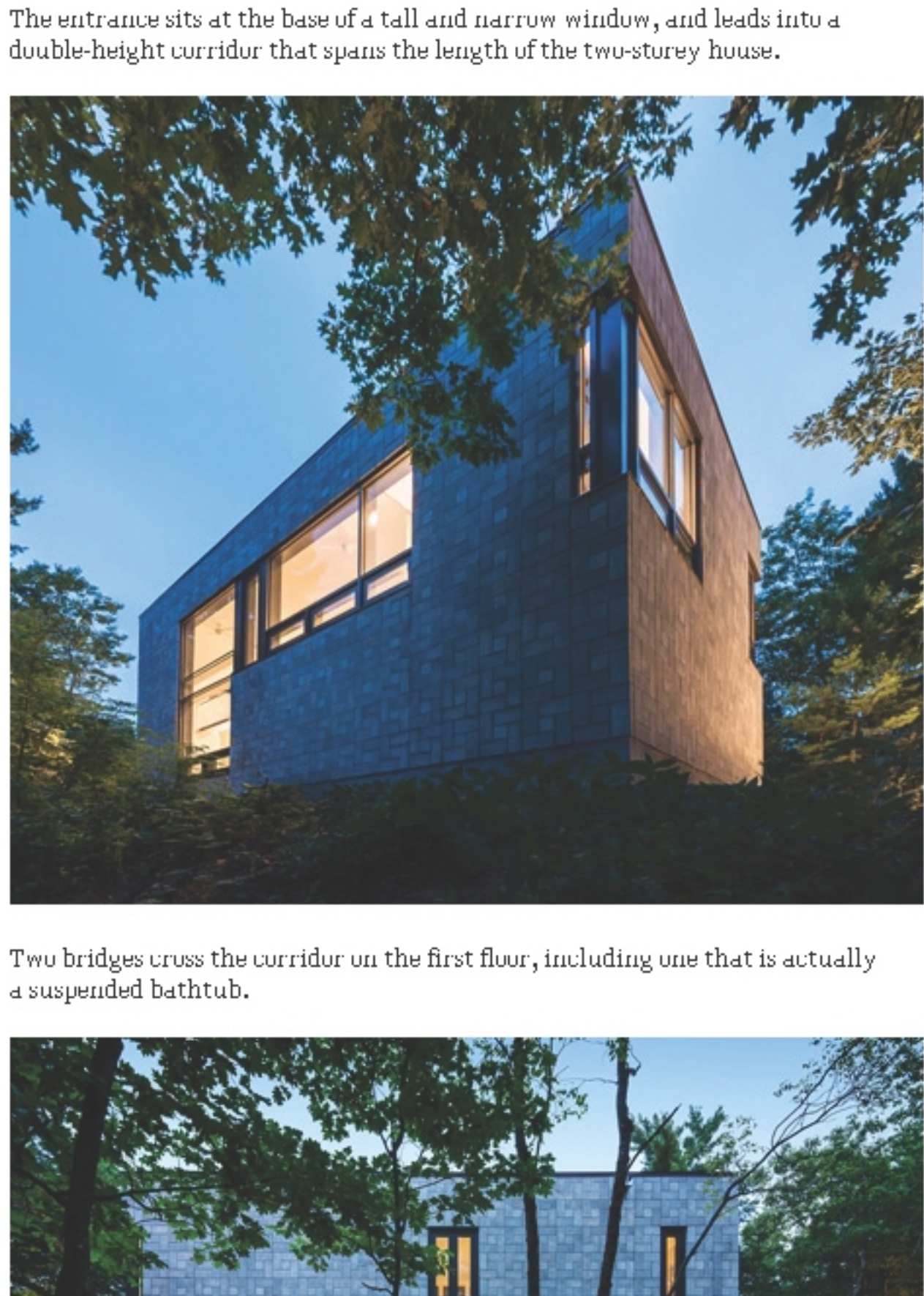
“We came up with this pattern by buying a stack of the blocks and just playing with them in the office,” DuBellet Kariouk told Dezeen . “The use of small and large blocks creates a more varied shadow pattern that also helps to break down the scale of the house.”
