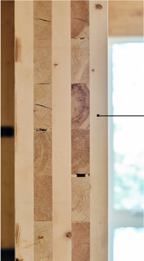
The exposed sections of cross-laminated timber — five-ply and just over seven inches thick — showcase the structure of the cottage
