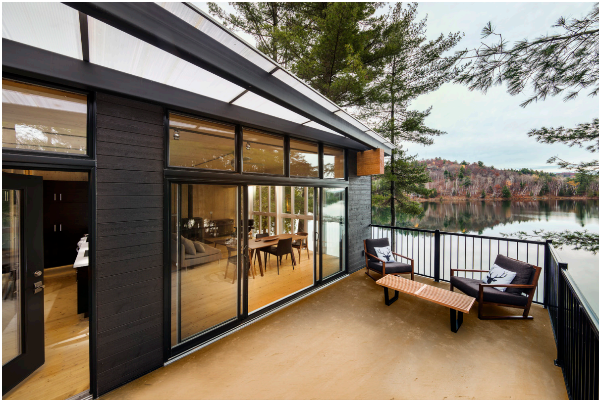
The new home is the same footprint of its now demolished predecessor, including an outdoor terrace that extends the interior great room courtesy of large sliding glass doors. PHOTOS:CHRISTIAN LALONDE, PHOTOLUX STUDIO
